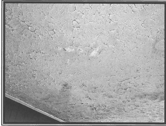
Photo #9 Asbestos-containing Stippled Ceiling Material in Room F
