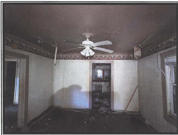
Photo #11 View Depicting Asbestos-containing Sheetrock Ceiling System in Room D
