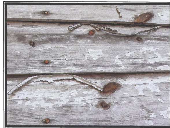
Photo #4 No Asbestos Detected in Caulk Associated with Wood Exterior Siding Planks
