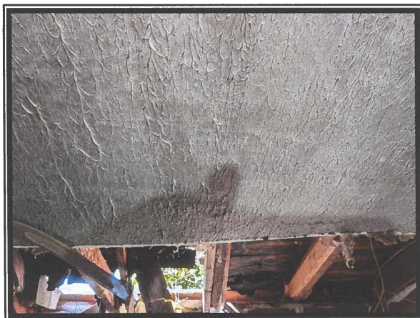
Photo #7 No Asbestos Detected in Stippled Ceiling Texture Material
