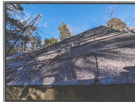
Photo #8 No Asbestos Detected in Roof Shingles of the Standalone Shed Structure
