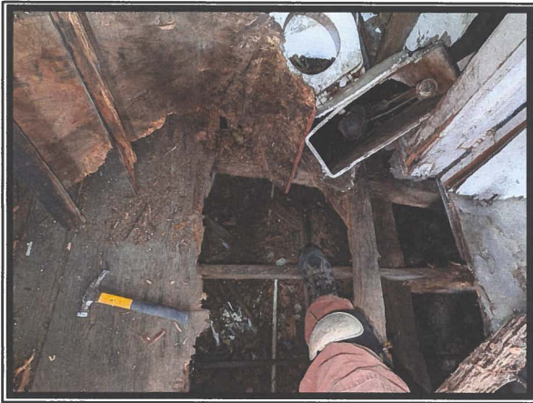
Photo #5 Asbestos-containing Sheet Flooring Observed under Collapsed Floor Area
