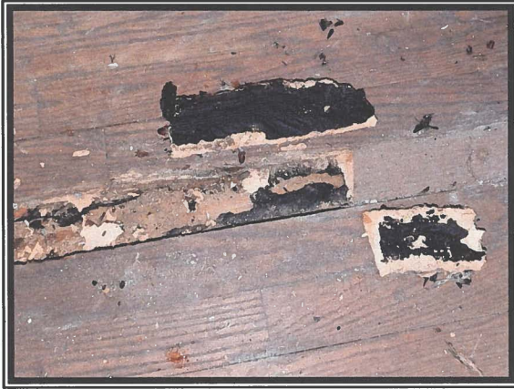
Photo #5 No Asbestos Detected in Flooring Vapor Felt Material
