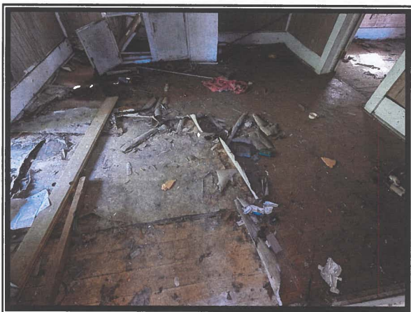
Photo #5 Asbestos Detected at 15% in Tan-colored, Bottom-layer Sheet Flooring in Room D
