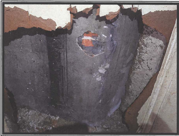
Photo #5 No Asbestos Detected in Surfacing Material on the Former Chimney Unit
