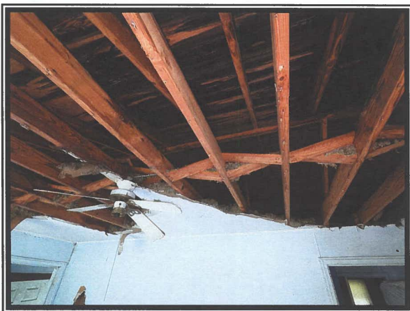
Photo #3 Asbestos Detected at 4% in Sheetrock Wall and Ceiling System
