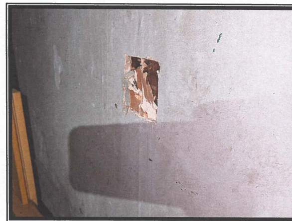
Photo #12 View Depicting Asbestos-containing Sheetrock Wall System in Room H
