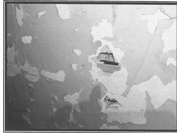
Photo #10 Asbestos-containing Plaster Wall over Wood Lath in Closet of Area (Hall) E
