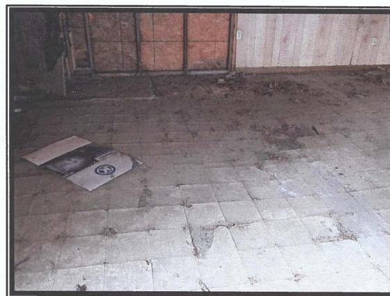
Photo #6 Asbestos Detected at 8% in 9x9 Floor Tiles of Area B
