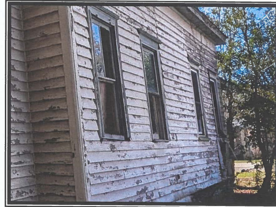
Photo #2 Asbestos Detected at 2% in Window Glaze Material
