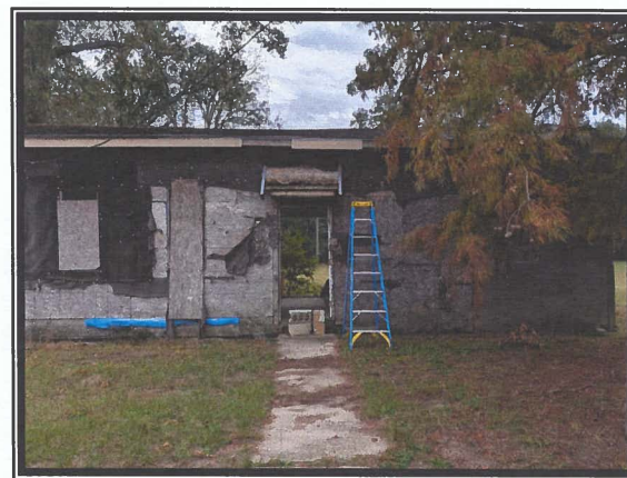
Photo #4 No Asbestos Detected in Remnant Felt Sheathing on Exterior Walls
