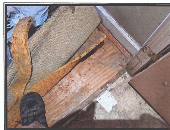
Photo #8 No Asbestos Detected in Sheet Flooring or Carpet Layers
