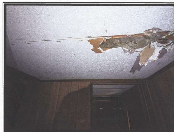
Photo #6 No Asbestos Detected in Ceiling Gypsum with Textured Surface Material
