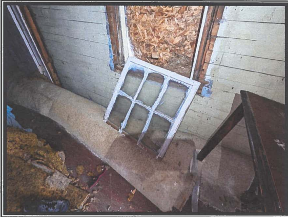
Photo #5 View Depicting Window Unit with Asbestos Detected in Glaze Material at >1%
