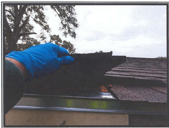
Photo #3 No Asbestos Detected in Roofing Shingles or Felt
