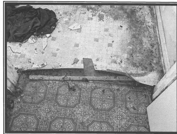
Photo #12 No Asbestos Detected in Any Resilient Sheet Flooring Layers
