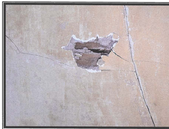
Photo #6 No Asbestos Detected in Plaster Wall System
