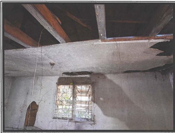
Photo #7 Asbestos-containing Stippled Ceiling Texture on Remnant Ceiling Surface
