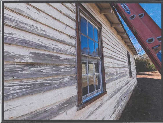
Photo #5 View Depicting Window Unit with Asbestos-containing Glaze Material
