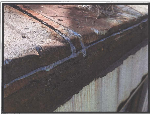
Photo #3 No Asbestos Detected in Roof Seam/Roof Edge Flashing Sealant
