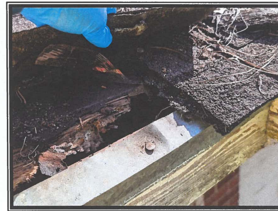
Photo #8 No Asbestos Detected in Roofing Shingles or Associated Felt Paper
