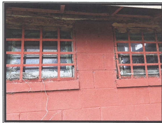
Photo #2 No Asbestos Detected in Window Pane Caulk of Restroom Windows
