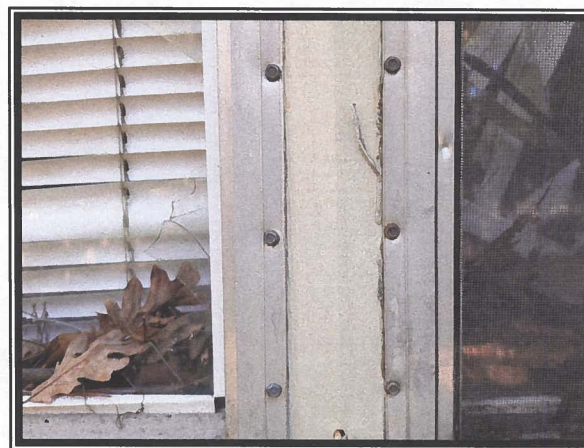
Photo #4 Asbestos Detected at 4% in Window Frame Caulk
