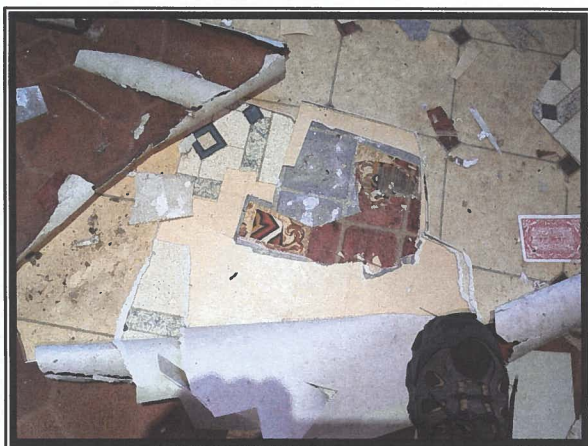
Photo #3 View Depicting Multi-layered Sheet Flooring with Asbestos-containing Layers in Room D
