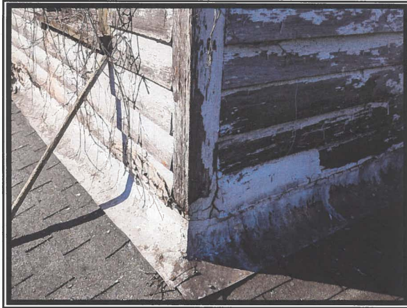
Photo #1 Asbestos Detected at 5% in Roof Flashing Sealant
