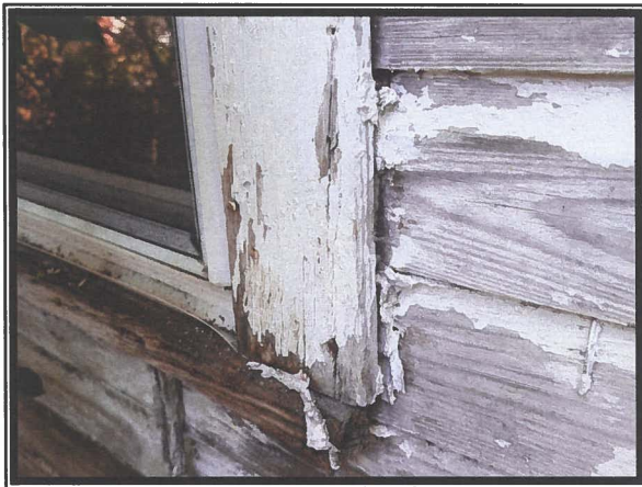
Photo #3 No Asbestos Detected in Window Frame Caulk
