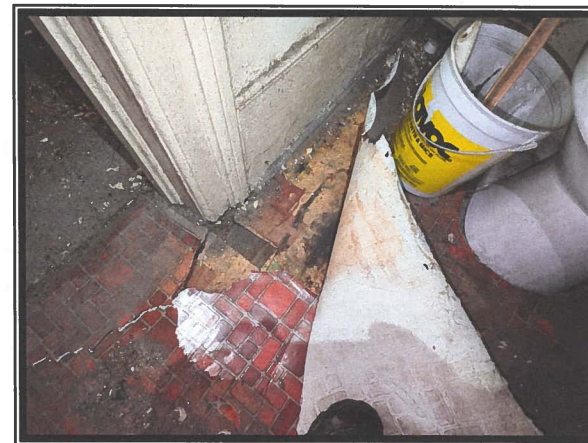
Photo #4 Asbestos Detected at 20% in Red, Small-brick Design Sheet Flooring in RR-2
