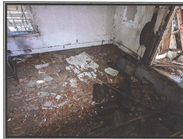
Photo #8 Asbestos-containing, Spray-applied & Stippled Ceiling Texture Scattered on Floors
