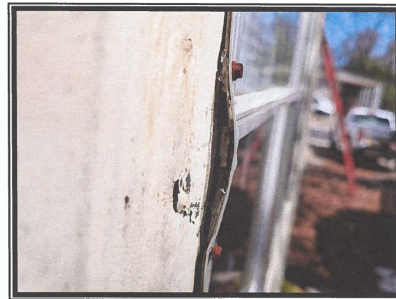
Photo #4 No Asbestos Detected in Window/Door Frame Caulk Material
