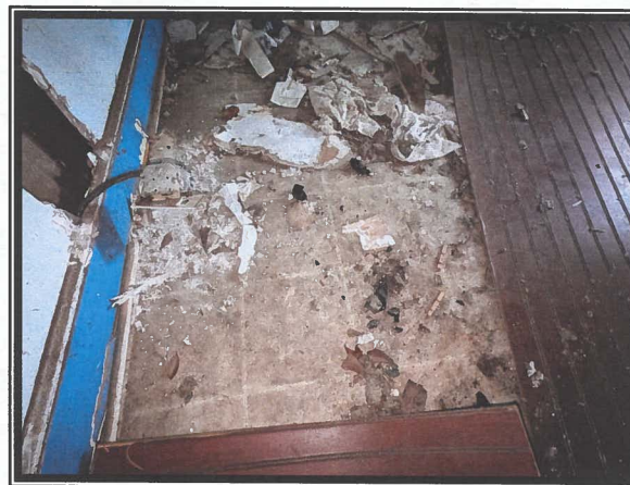
Photo #6 No Asbestos Detected in Sheet Flooring in Kitchen Area
