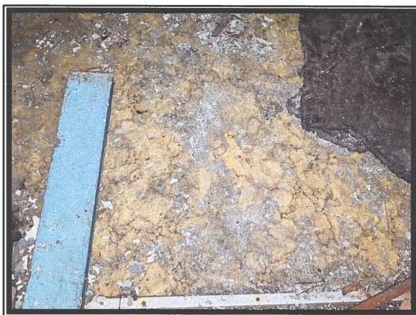
Photo #5 Asbestos Detected at 20% in Mottled Yellowish Tan Sheet Flooring in Room 1C
