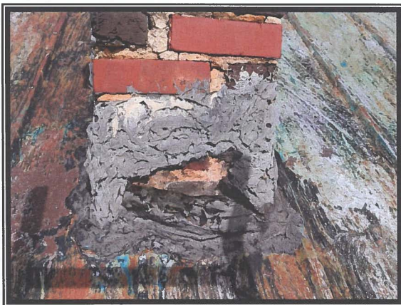
Photo #3 Asbestos Detected at >1% in Chimney and Roof Ridge Sealant Material
