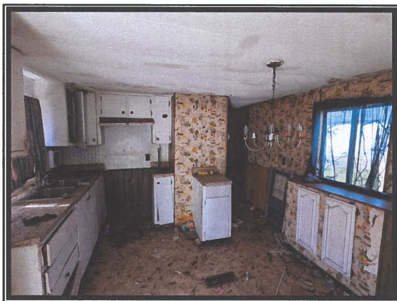
Photo #5 No Asbestos Detected in Wallpaper Layers
