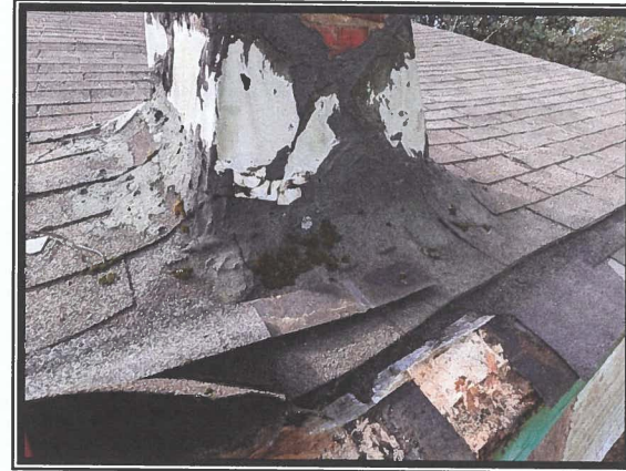
Photo #2 Asbestos Detected at 3% in Chimney Flashing Sealant Material
