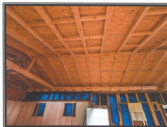
Photo #8 View Depicting Uncovered, Wood-framed Ceiling/Roof Structure
