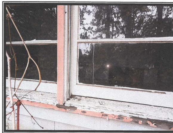
Photo #2 Asbestos Detected in Window Glaze Material at <0.19%
