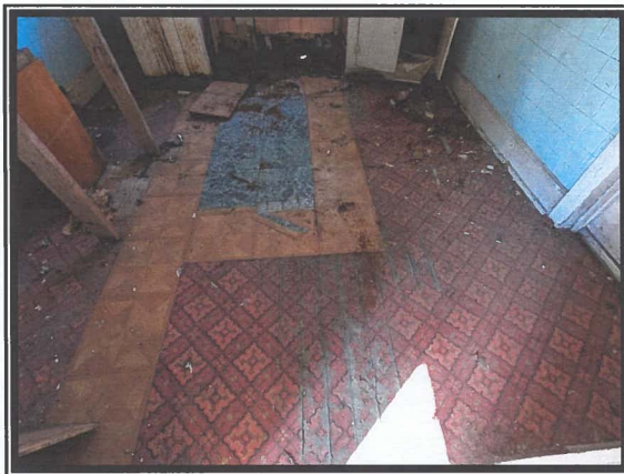
Photo #3 Asbestos-containing, Red-colored Sheet Flooring in Room C
