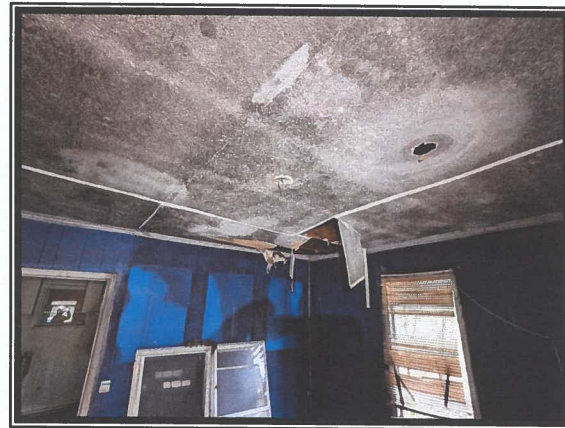
Photo #4 Spray-applied Texture over Sheetrock Ceiling in Room A - No Asbestos Detected
