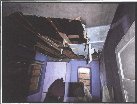
Photo #7 Significantly Damaged Sheetrock Ceiling in Room C - No Asbestos Detected
