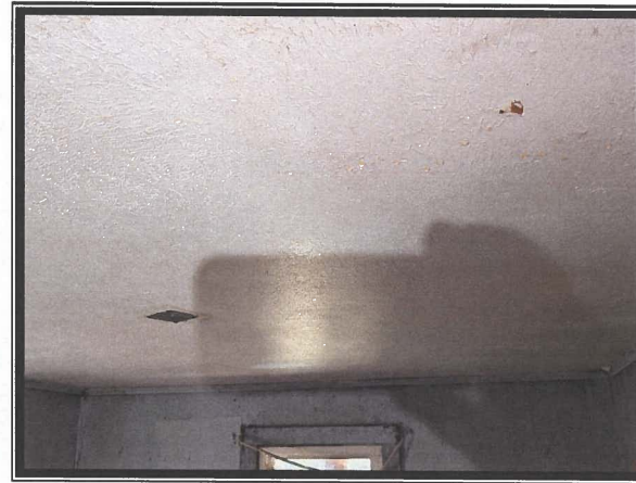
Photo #6 Asbestos Detected at Less than 1% in Stippled Ceiling Texture of Room H
