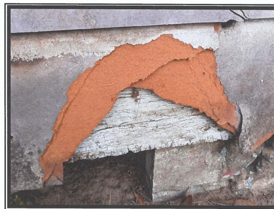
Photo #6 No Asbestos Detected in Cellulose-based Exterior Siding Material
