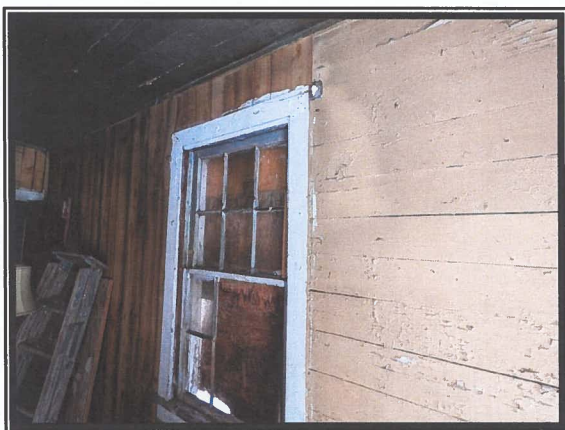
Photo #7 View Depicting Wood Paneling over Wood Slat Interior Walls
