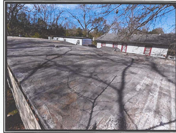
Photo #2 Asbestos Detected at 1.7% in Silver Roof Sealant Material
