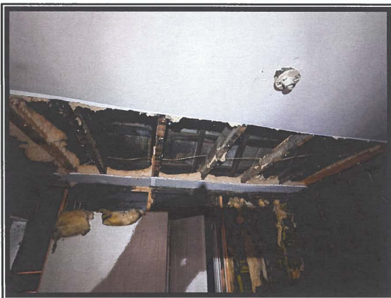
Photo #7 No Asbestos Detected in Sheetrock Ceiling System
