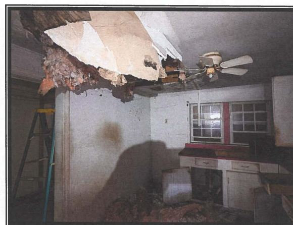
Photo #4 Asbestos-containing Sheetrock Ceiling System in Room G
