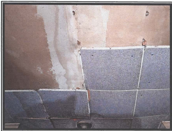
Photo #7 Fiberboard Ceiling Tiles attached to Asbestos- containing Sheetrock Ceiling System
