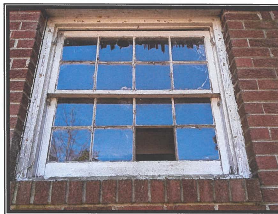
Photo #2 Asbestos Detected at 3% in Window Frame Caulk (<0.11% Detected in Window Glaze)
