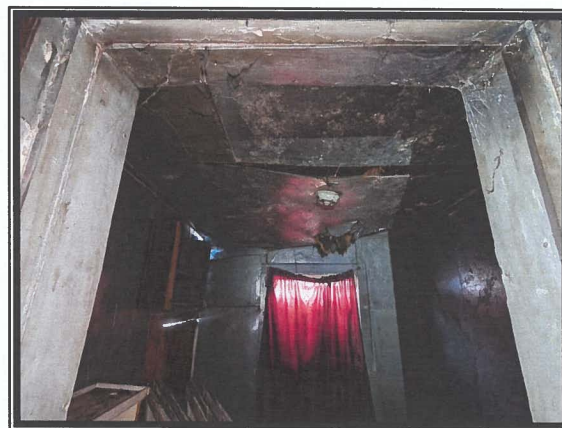
Photo #10 No Asbestos Detected in Cellulose-based Ceiling and Wall Panels in Room D
