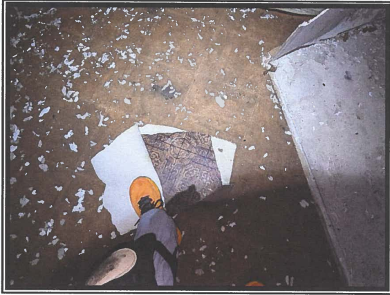
Photo #5 Two Layers of Sheet Flooring in Room B - No Asbestos Detected
