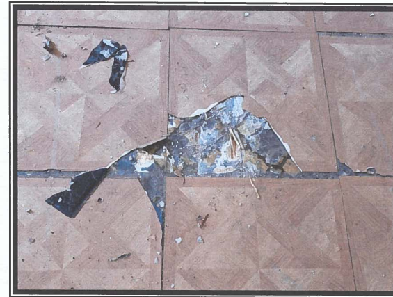
Photo #2 Asbestos-containing, Mottled Green Flooring under Parquet-design Squares in Rm. B
