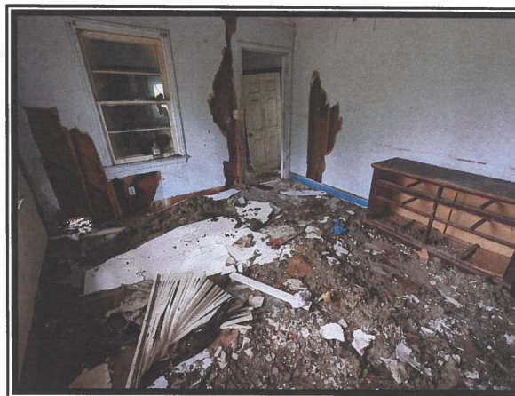
Photo #4 View Depicting Asbestos-containing Sheetrock Debris on Floor of Room A
