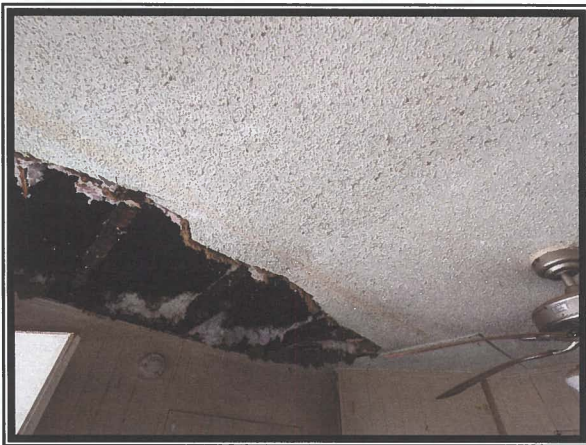
Photo #7 No Asbestos Detected in Spray-applied Ceiling Texture
