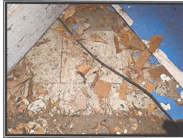
Photo #6 Asbestos Detected at 5% in Various 9x9 Floor Tile Types
