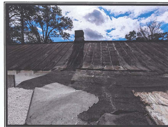
Photo #4 No Asbestos Detected in Roof Shingle Rolls or Associated Felt Paper
