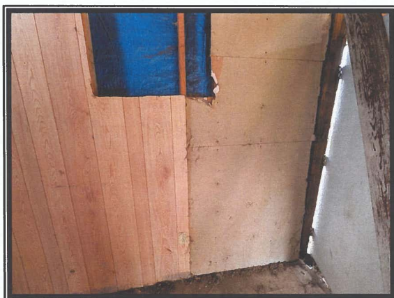
Photo #7 No Asbestos Detected in Gypsum Wall Panels Located in Area B
