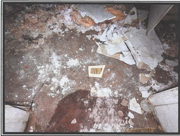
Photo #9 Asbestos-containing Sheetrock Materials Scattered on Floor in Room G
