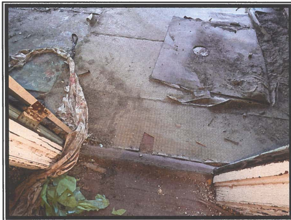
Photo #3 Asbestos Detected at 15% in Tan Sheet Flooring with Red Designs in Room 2C
