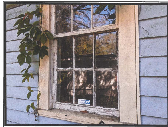
Photo #4 No Asbestos Detected in Window Units' Sealant Caulk
