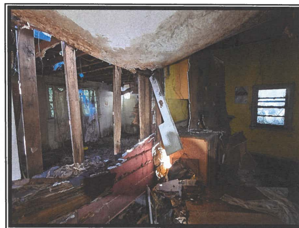
Photo #4 View Depicting Collapsed and Hazardous Interior Conditions
