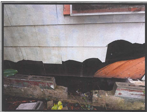
Photo #1 Asbestos Detected in Transite Siding at 10%; Asbestos Detected in Wall Felt at <0.1%
