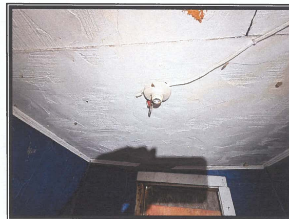
Photo #8 No Asbestos Detected in Cellulose-based Ceiling and Wall Panels of the Restroom Area
