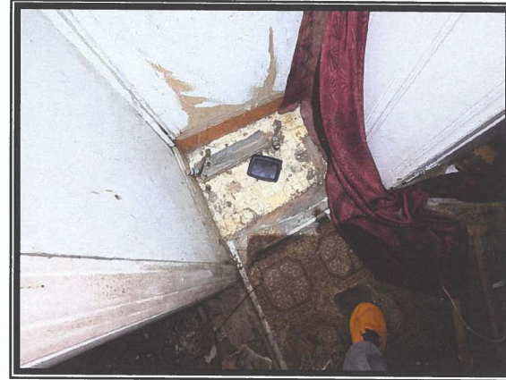
Photo #6 Asbestos Detected at 30% in Bottom-layer, Yellowish Tan Sheet Flooring in Room F
