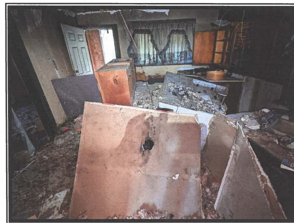
Photo #8 No Asbestos Detected in Sheetrock Systems Associated with Ceilings or Walls
