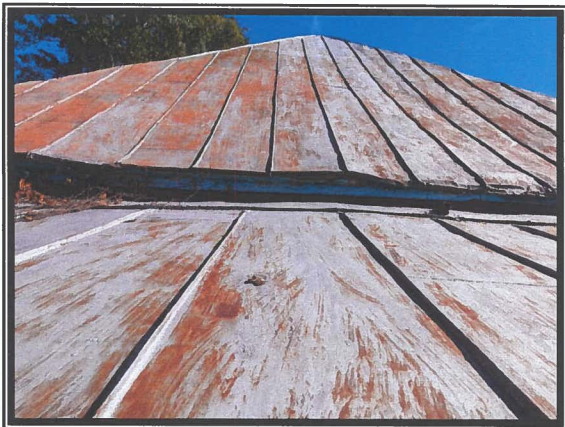
Photo #3 Asbestos Detected at 2% in Silver Sealant Associated with Sheet Metal Roof Panels
