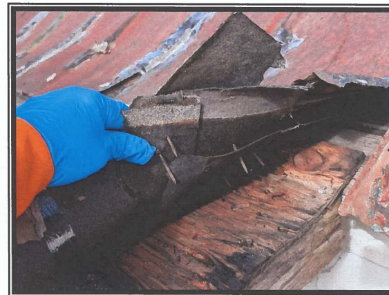
Photo #4 Asbestos Detected at <1% in Felt Paper Associated with Shingled Roof Area
