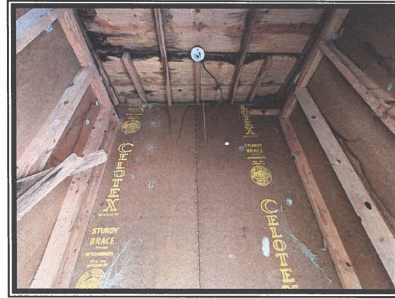
Photo #6 No Asbestos Detected in Celotex Wall Sheathing Panels
