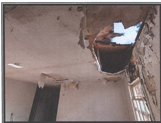
Photo #3 Asbestos Detected in Sheetrock System at 3% & in Spray-applied Ceiling Texture at 2%
