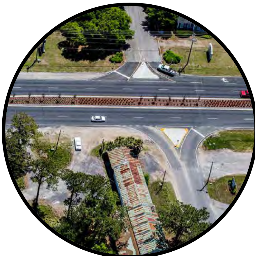
Access Management/ Median Break Closures
