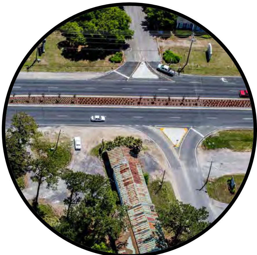
Access Management/ Median Break Closures
