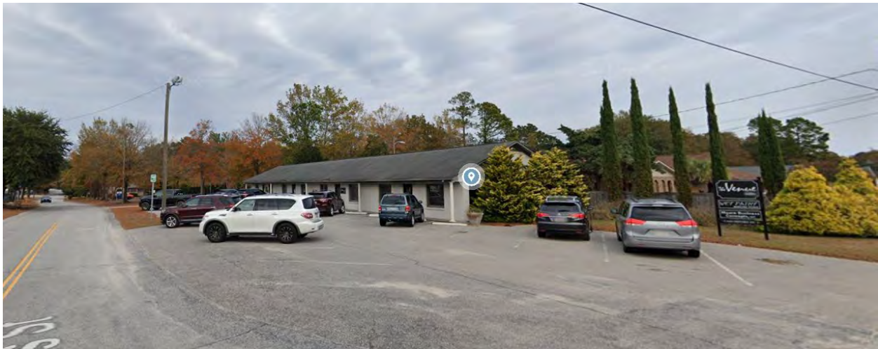
Above: Picture of subject property from intersection of Oxford St. and Willis St. Source: November 2023 Google Streetview Imagery
