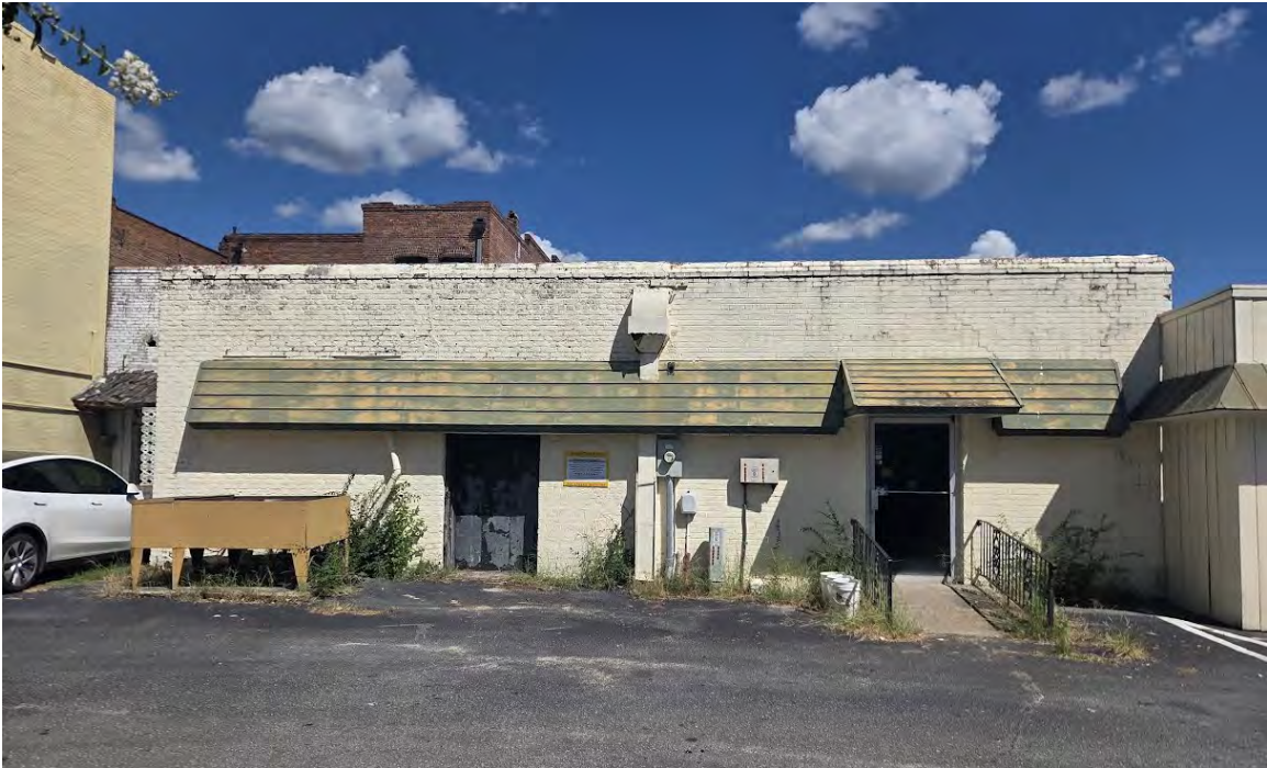
Figure 4 – Rear Façade of Building
