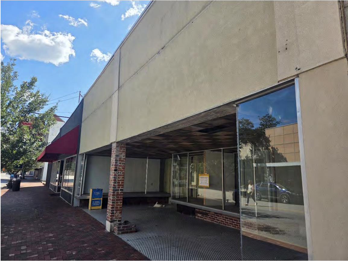
Figure 3 – Front Façade of Building
