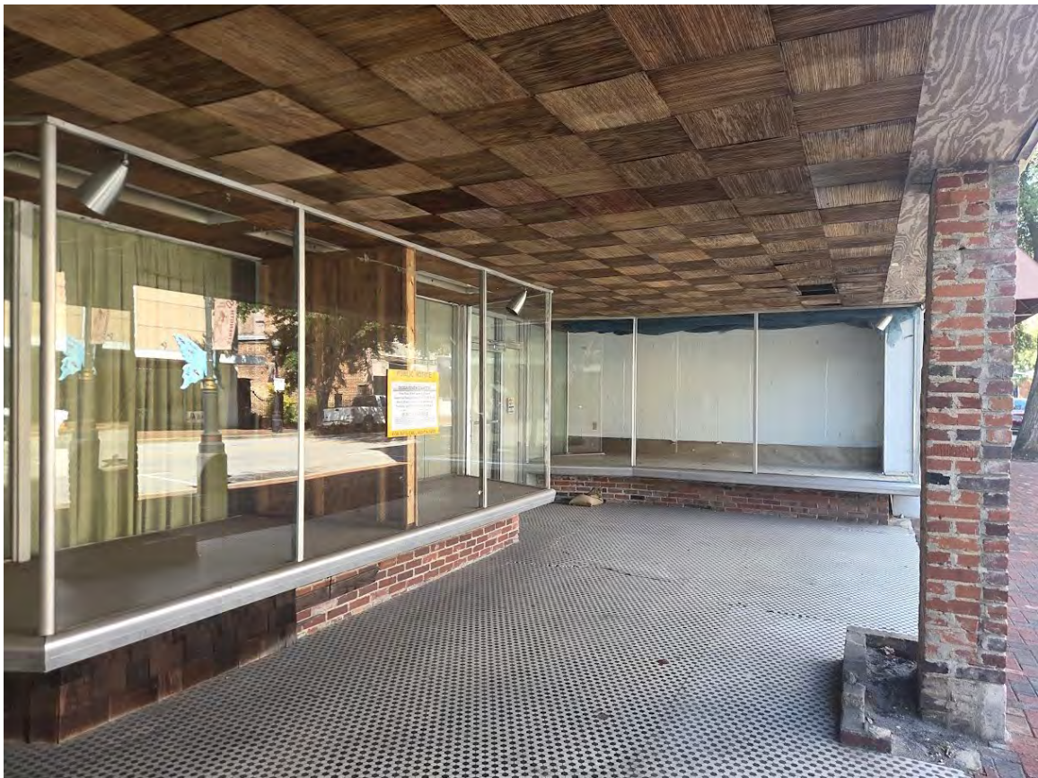
Figure 6 – Recessed Storefront of Building facing N. Main St.
