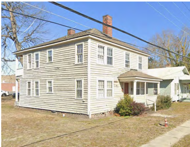
West-facing side of residence as viewed from Dugan St.
