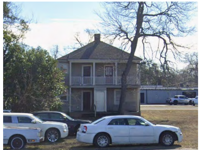
Site rear (north-facing) as viewed from Liberty St.
