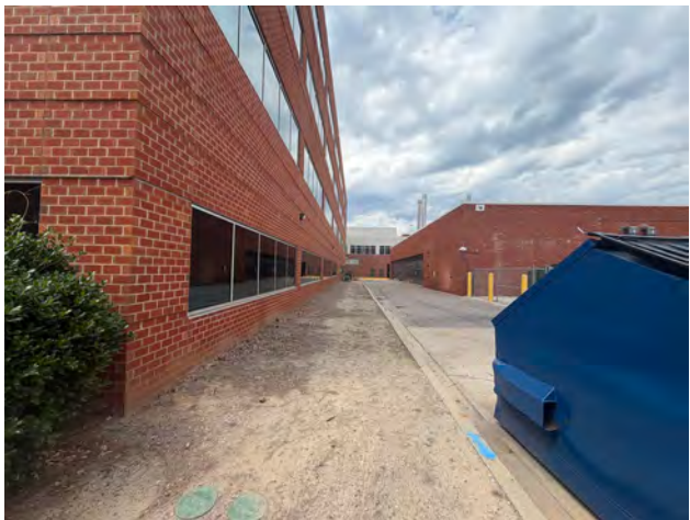
Above: Alleyway where the storage tank will be located
