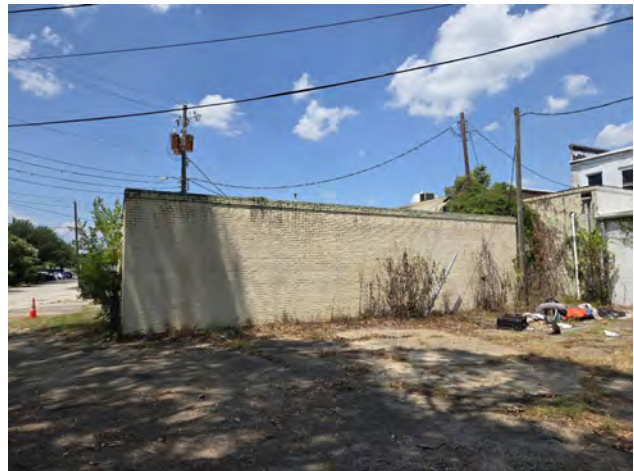
Above: Subject building, as viewed from south
