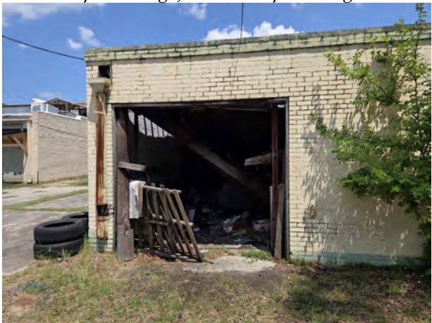
Above: Subject building, as viewed from rear
