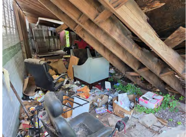
Above: Subject building interior
