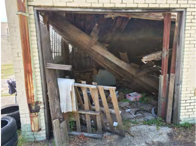
Above: Subject building interior, as viewed from rear garage door opening.
