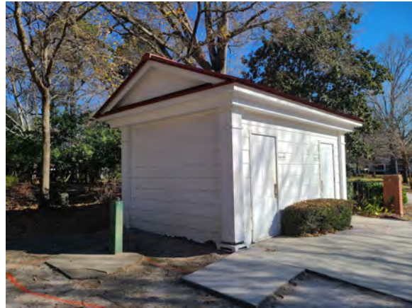
Above: Existing park restroom building (side view)
