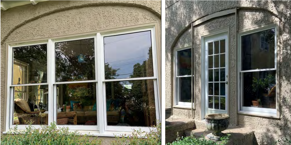
Above: Current porch windows and porch door configuration
