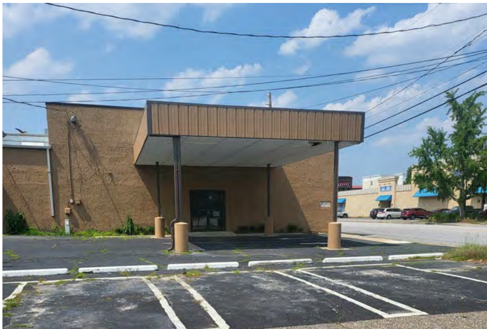
Above: View of the building and Porte cochere, prior to commencement of work.
