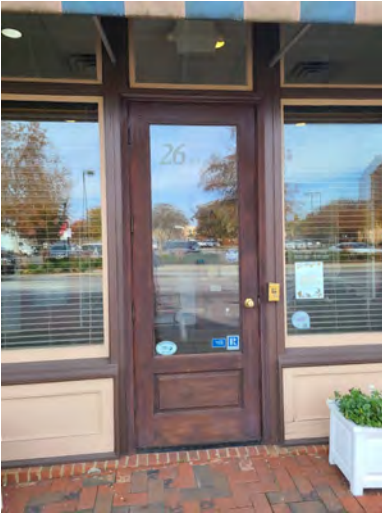
Existing Front Door
