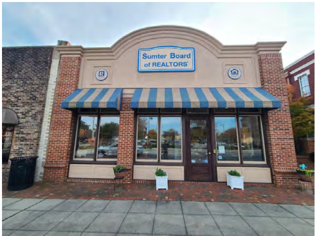
Above: 26 E. Liberty St. front facade as viewed from E. Liberty St.
