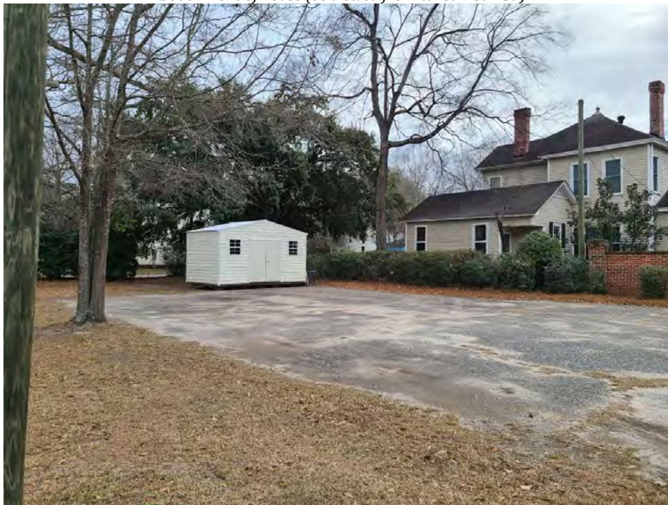
Above: Accessory Building as viewed from W. Calhoun St.
