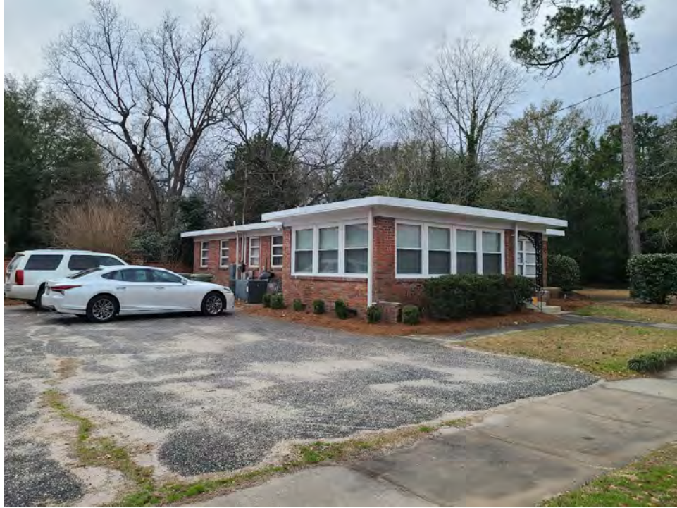
Above: Front of house (as viewed from W. Calhoun St.)
