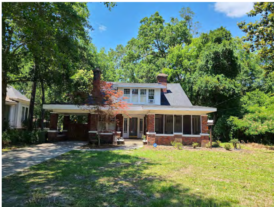
Above: Front of house (as viewed from W. Hampton Ave)
