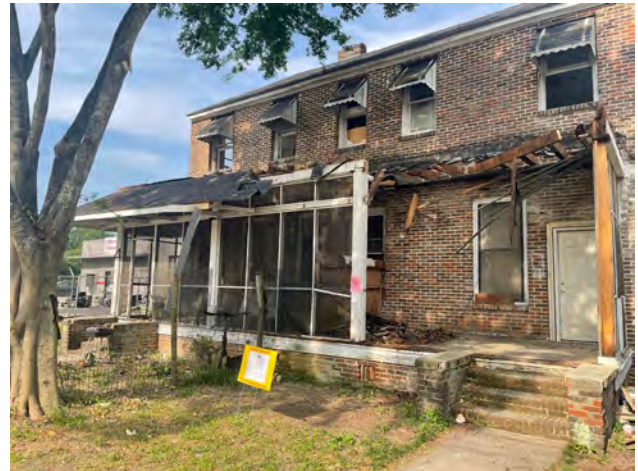
Site Front as viewed from Church St.
