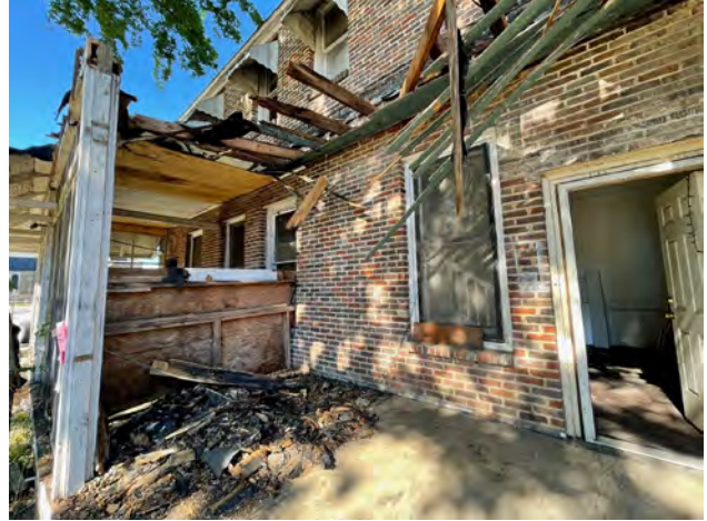
Partial Demolition prior to Stop Work Order
