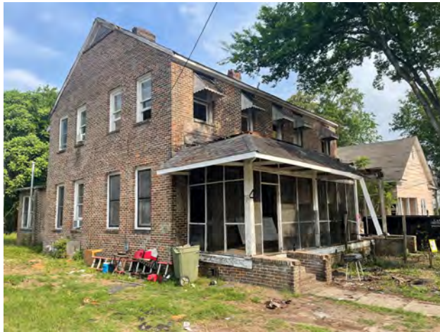
Site Front as viewed from Church St.
