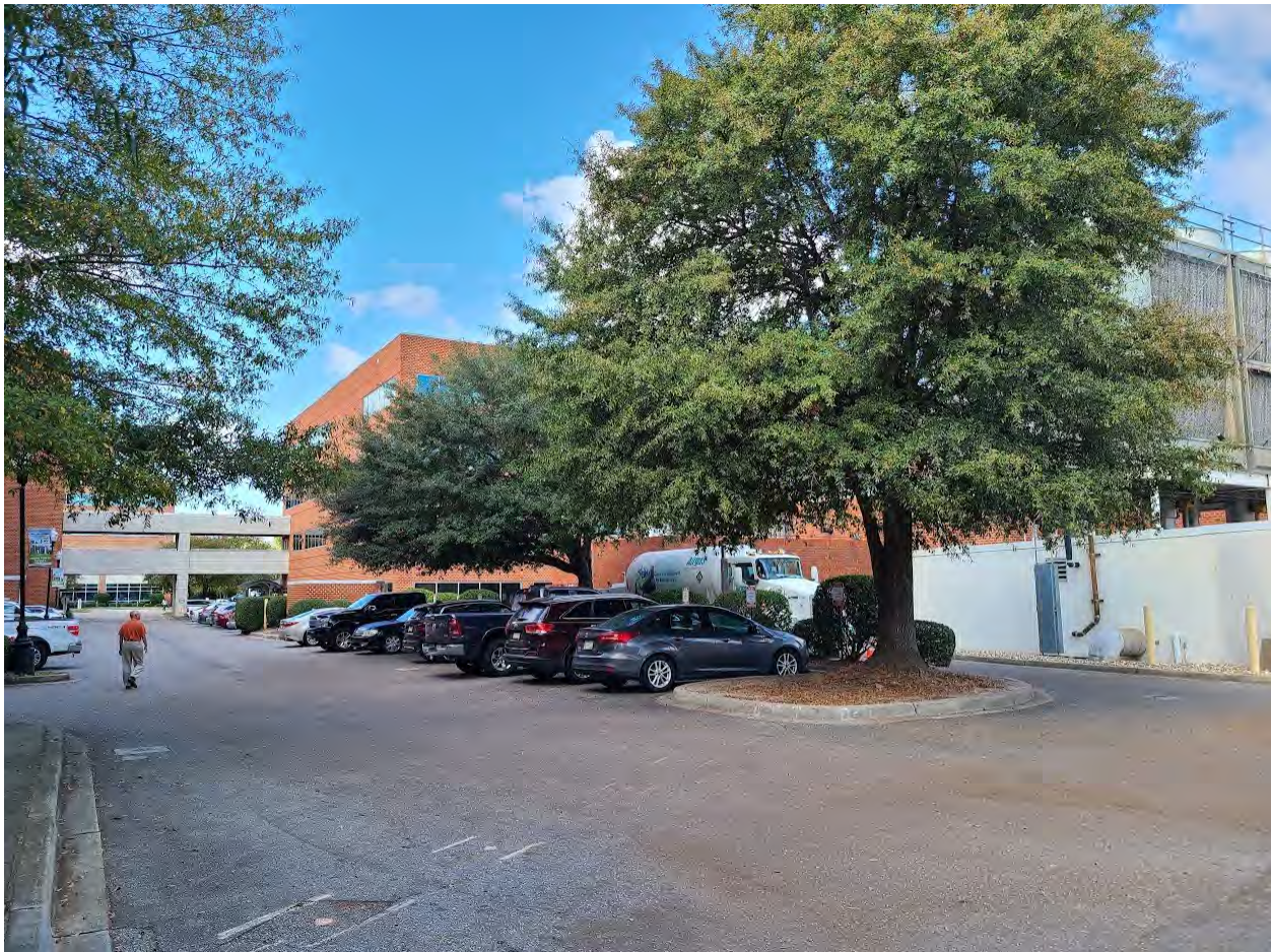
Above: View of the existing trees and parking area where generators are proposed for installation
