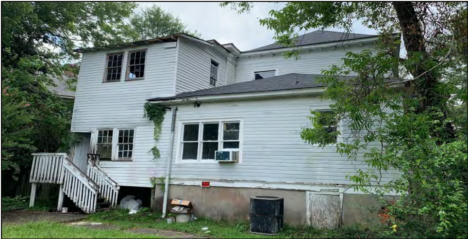
Above: rear view of residence prior to alterations approved via HP-19-13 showing previous 1 st floor rear access stair configuration and covered 2 nd floor addition that has been modified.
