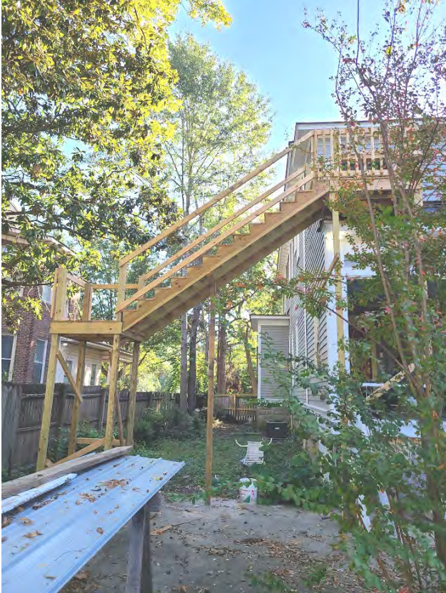
Above: Partially constructed staircase as viewed from rear.
