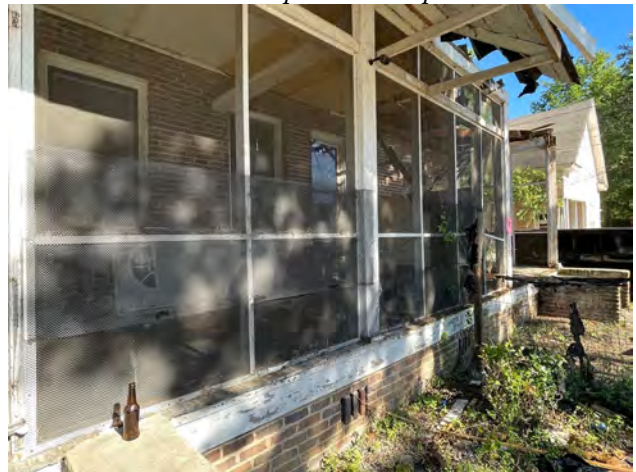
Screen Deterioration
