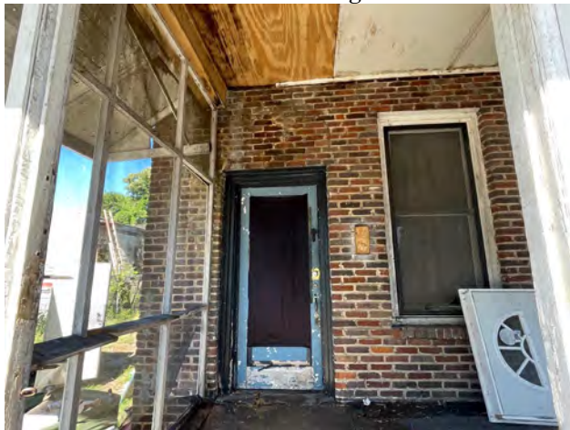
Ceiling Deterioration
