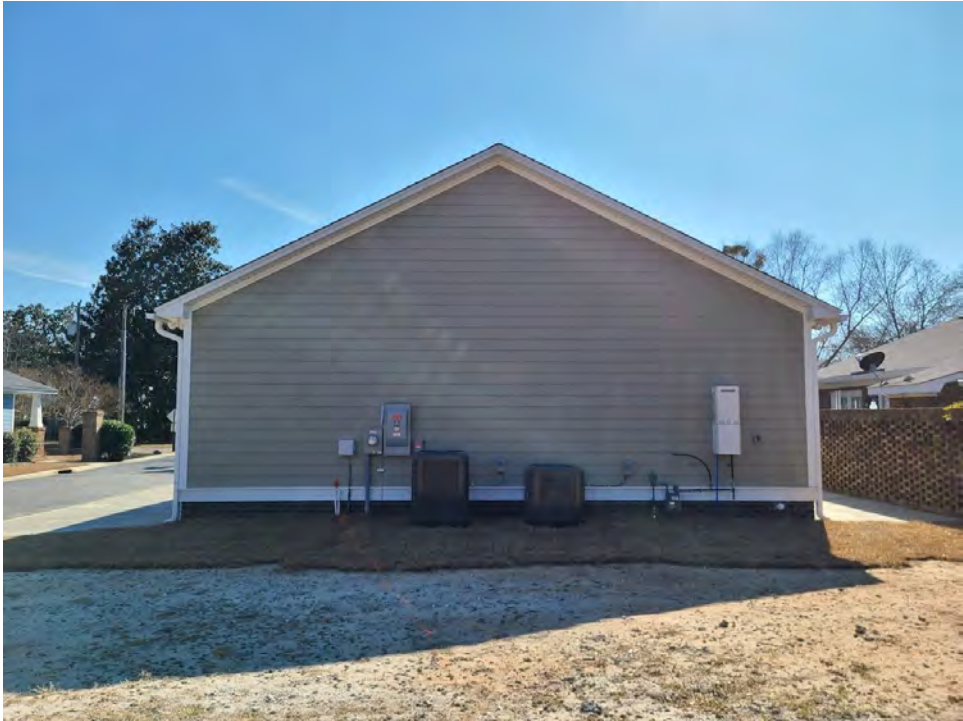
The rear elevation (above) continues with horizontal lap siding.
