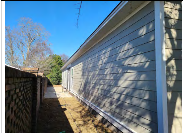
West façade of 80 Calhoun Pl.
