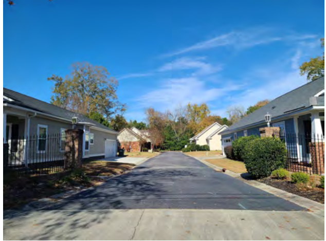
View from W. Calhoun St. toward rear of development.
