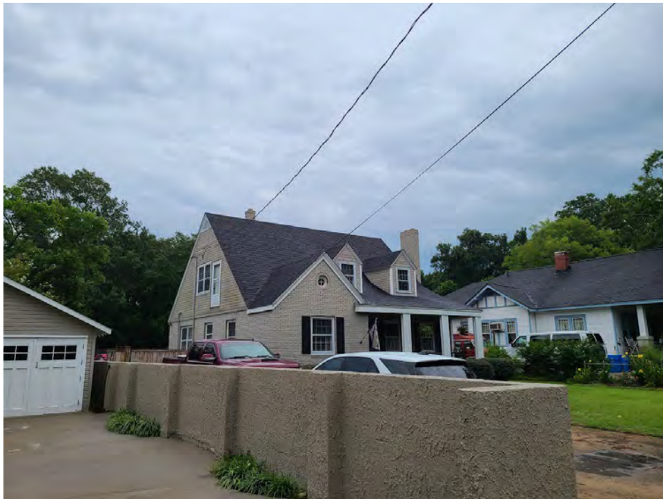
Above: Property as viewed from north (as viewed from McQueen St.)
