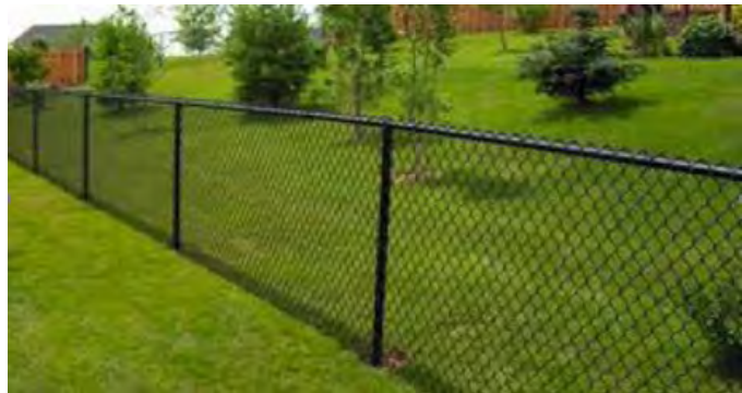
6 ft. Black Vinyl Chain-link Fence (typical)
