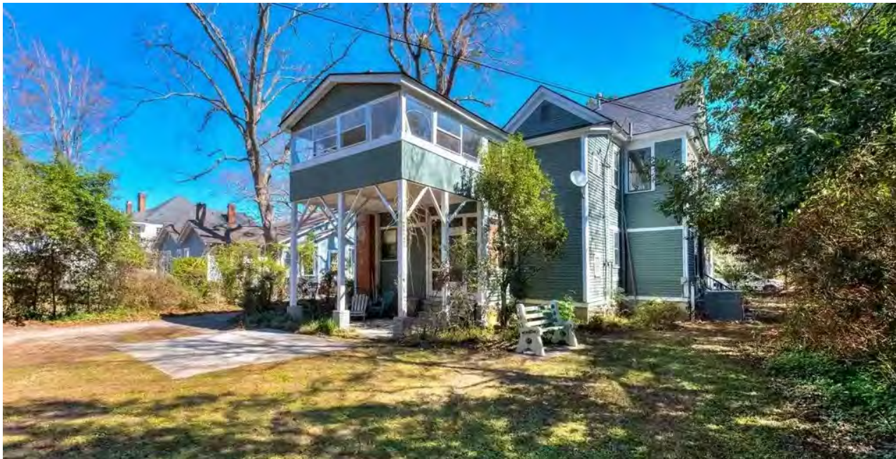
Above: Rear View of 24 Park Ave. Pictured: HVAC and Proposed Location for Dog Pen
