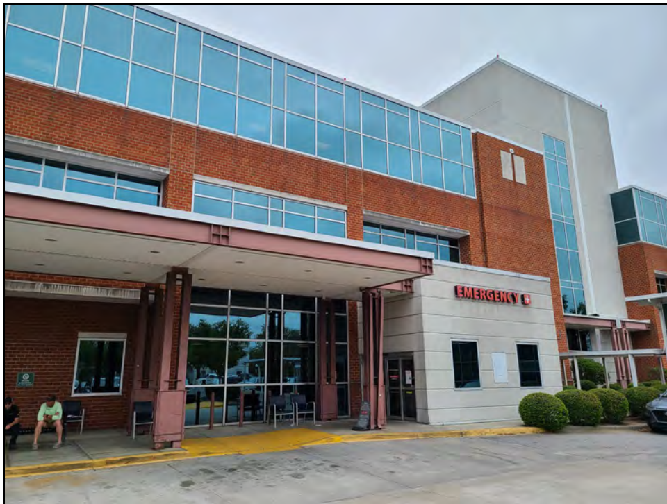
Above: View of the existing emergency room front (N. Main St. façade)
