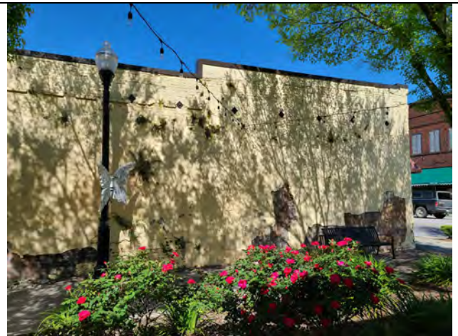
36 W. Liberty St. (Osteen Publishing Co./Sumter Item east-facing wall)
