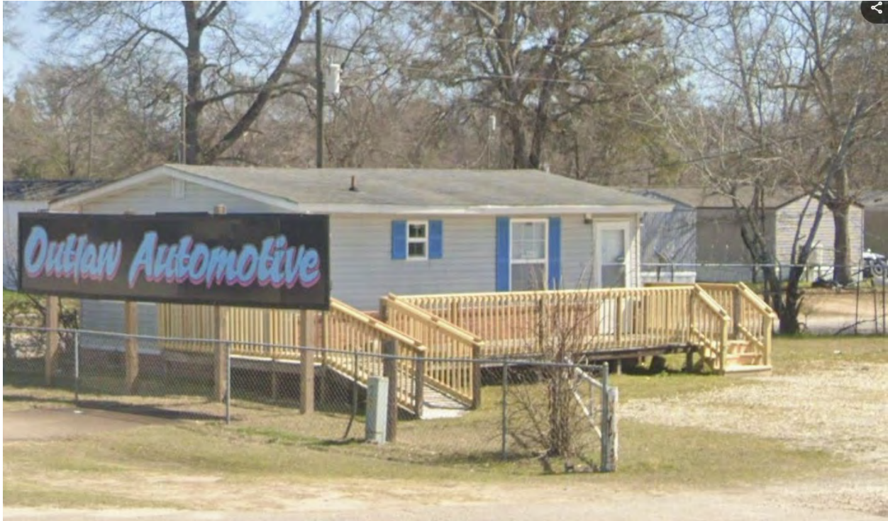
Above: Subject building as viewed from Broad St.
