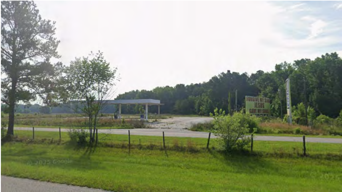
Figure 2 - Site Conditions (as of 2025)
