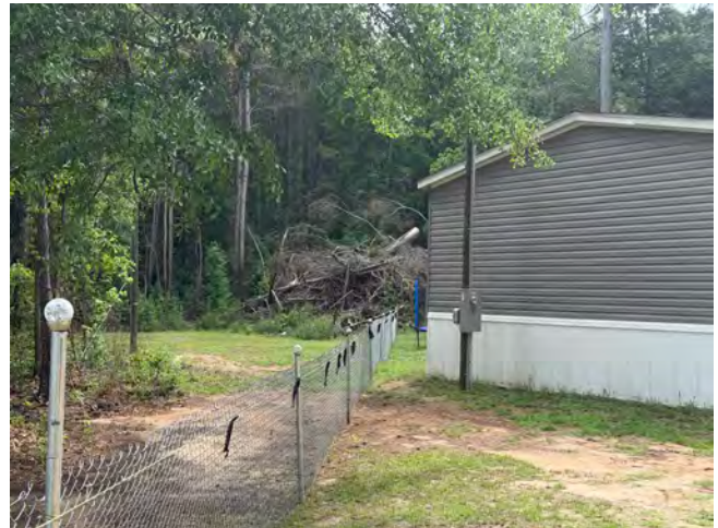
Figure 3: View of property line specifically highlighting placement of mobile home relative to the property line
