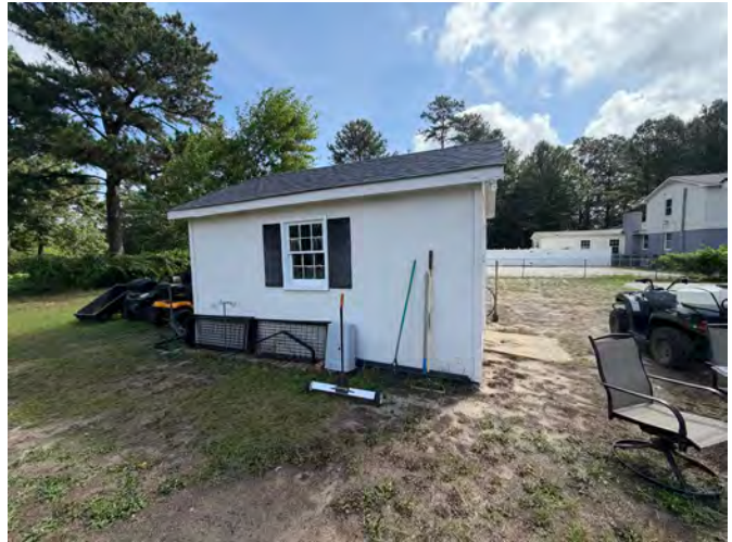
Figure 3: Existing accessory structure to be removed
