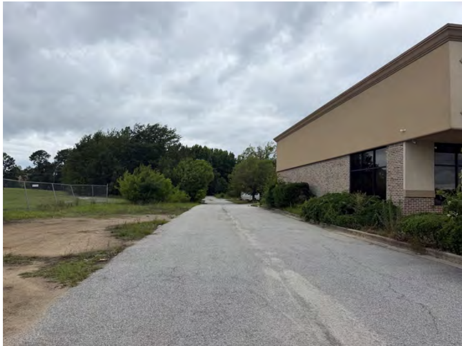
Figure 2 – Entrance off Wesmark Blvd.) (June 2026)
