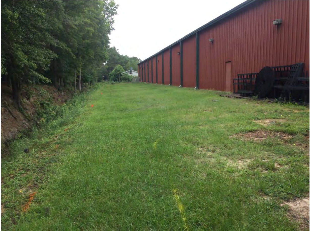
Figure 2: Existing conditions of proposed location
