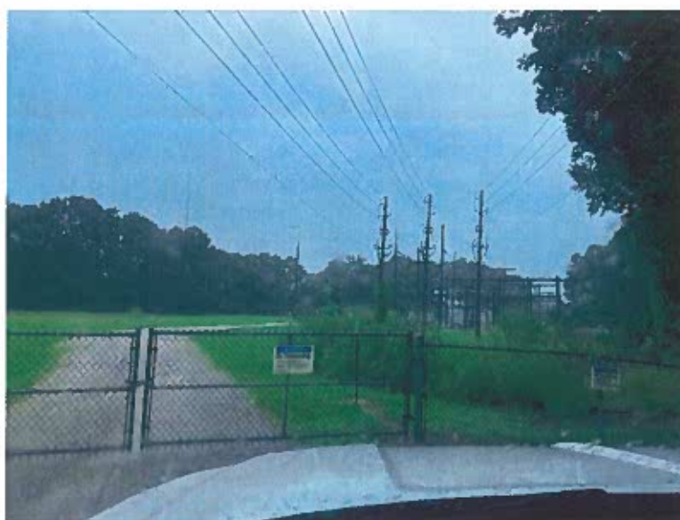
Figure 2: Photo of existing conditions at Alice Dr.
