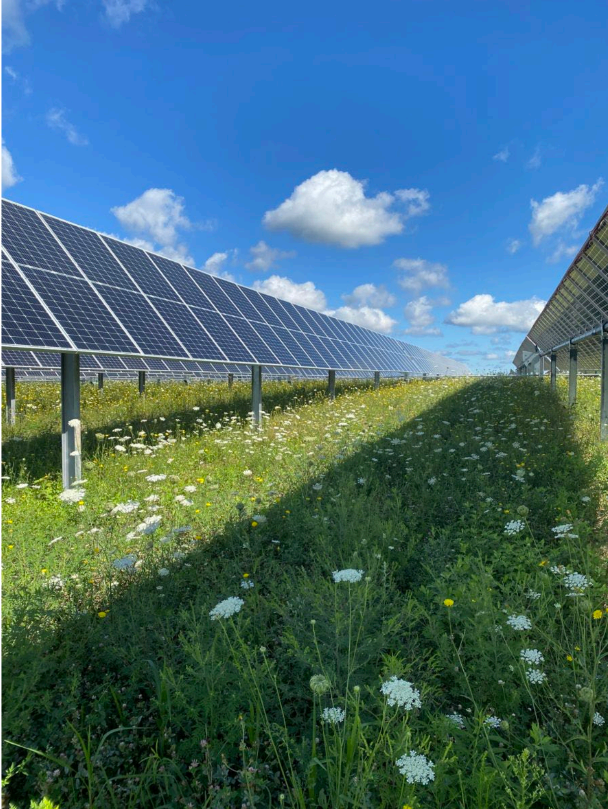
Figure 2. Single-axis, tracking solar PV array with panels near maximum tilt as viewed from the east or west
