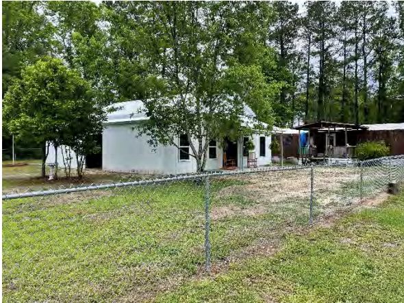
Figure 1: East Side View
