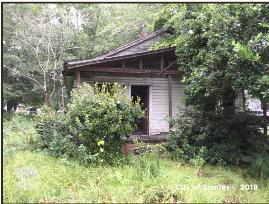
Photograph 14 Crosswell Example of "Hazard" Condition Property
