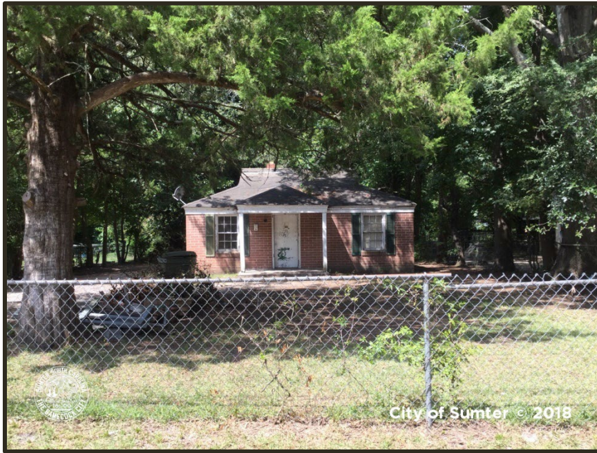
Photograph 32 Magnolia-Harmony Example of "Poor" Condition Property
