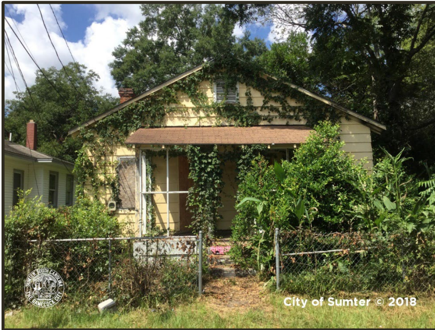
Photograph 47 Savage Glover Example of "Poor" Condition Property
