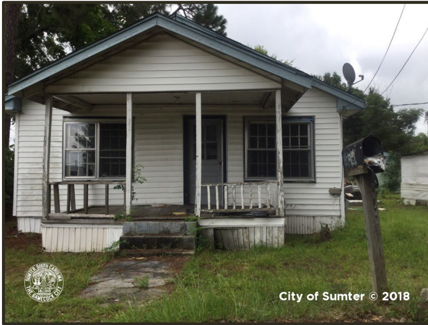
Photograph 48 Palmetto Park Example of "Poor" Condition Property
