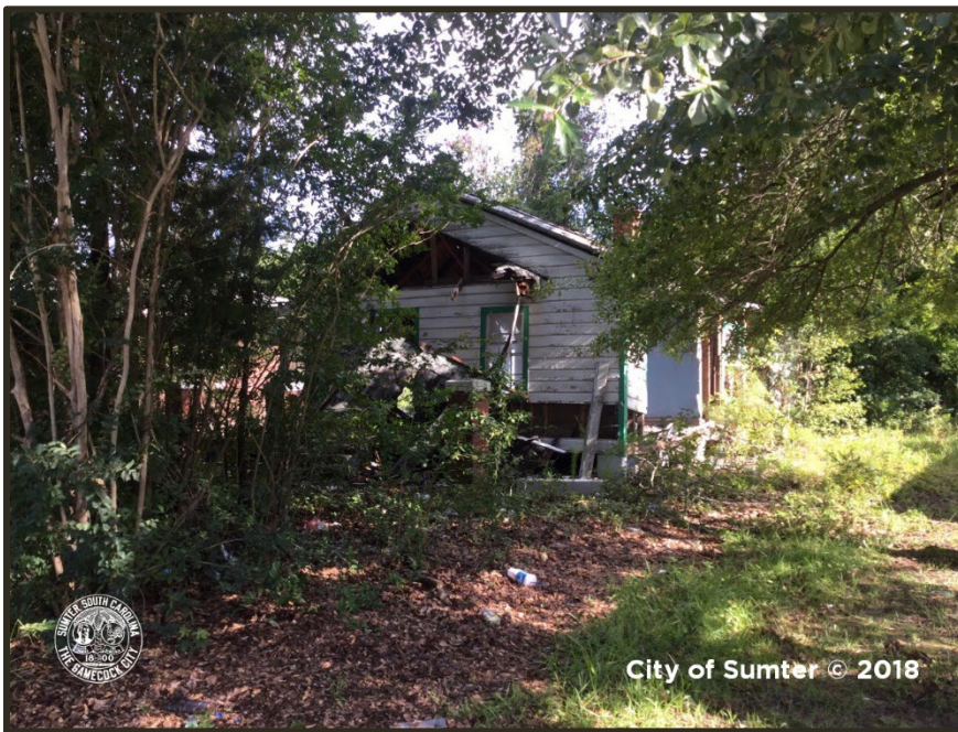
Photograph 42 Mulberry Example of "Hazard" Condition Property
