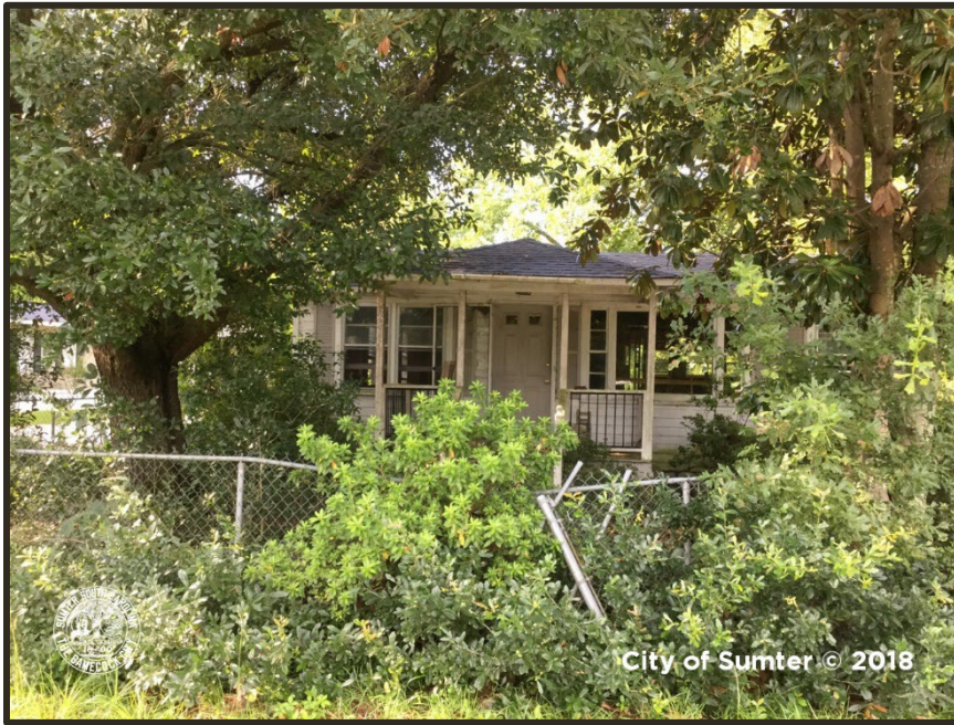
Photograph 41 Mulberry Example of "Poor" Condition Property
