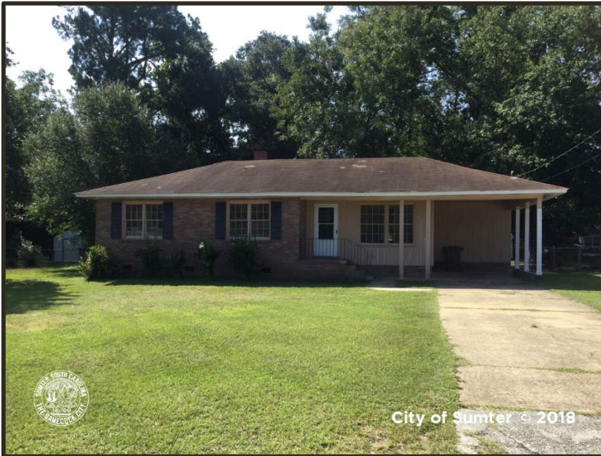
Photograph 34 Millwood Example of "Good" Condition Property
