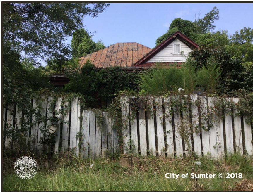
Photograph 59 South Liberty Example of "Hazard" Condition Property
