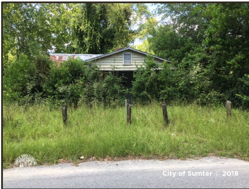
Photograph 63 Swan Lake Example of "Hazard" Condition Property
