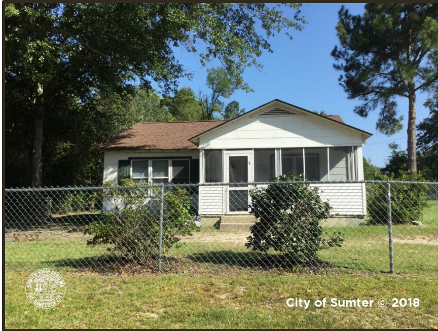
Photograph 22 Lemira Example of "Good" Condition Property
