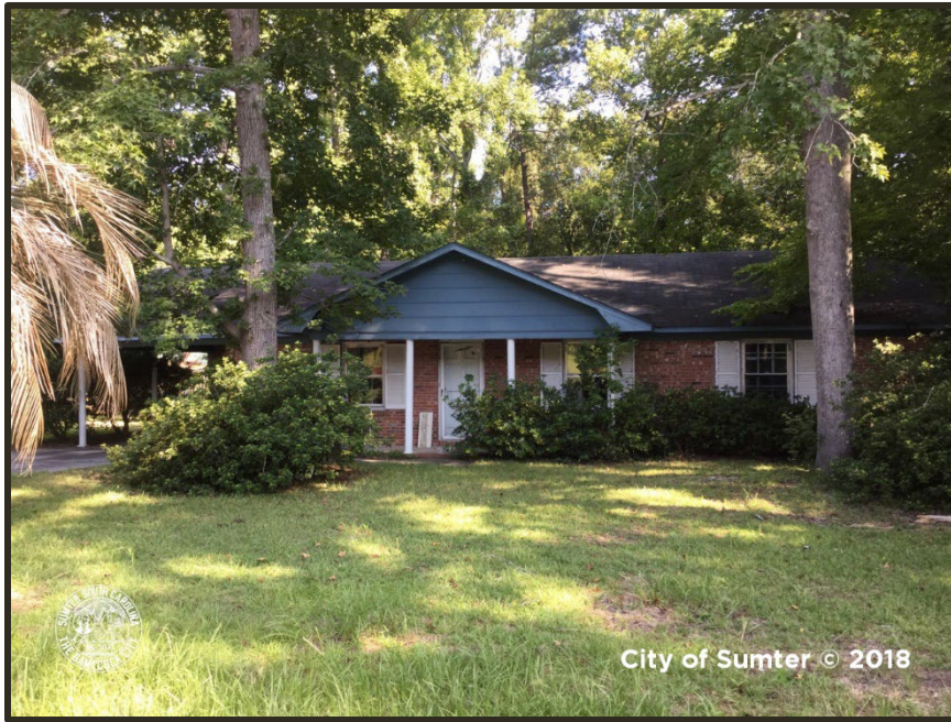
Photograph 367 Millwood Example of “Hazard” Condition Property
