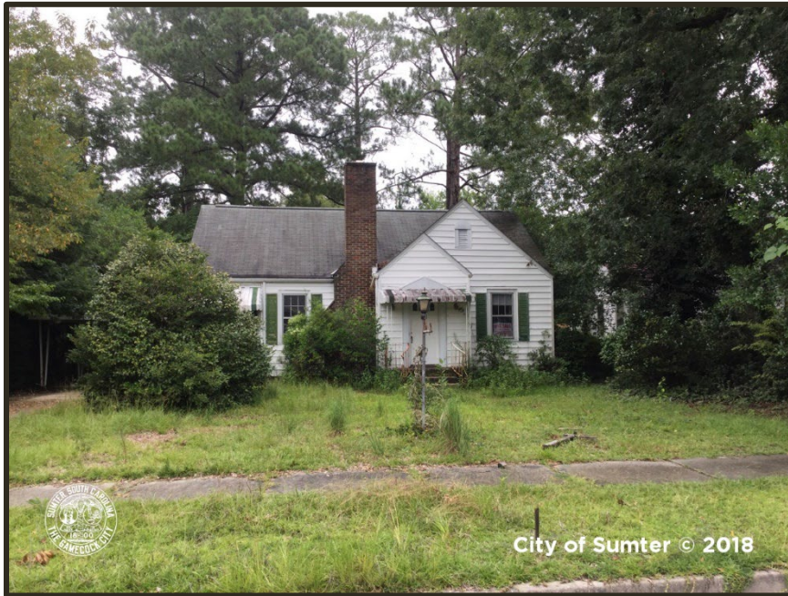
Photograph 13 Crosswell Example of "Poor" Condition Property
