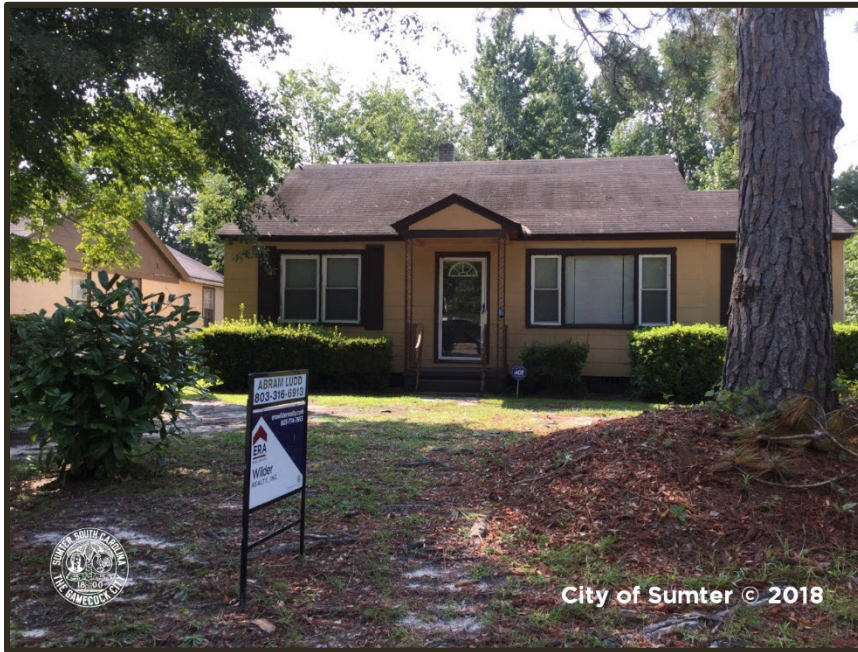
Photograph 11 Crosswell Example of "Good" Condition Property
