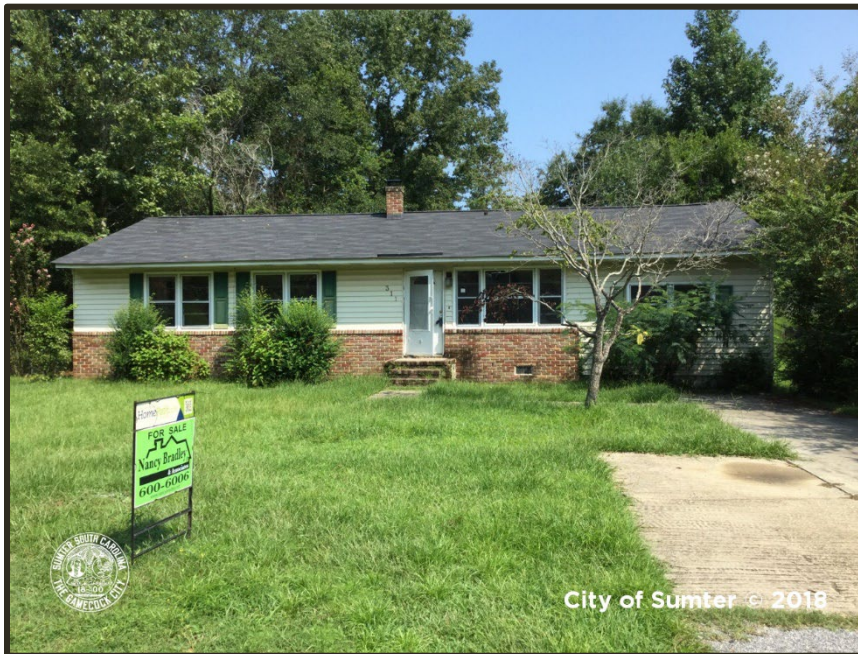
Photograph 12 Crosswell Example of "Fair" Condition Property
