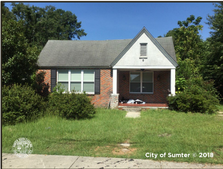
Photograph 20 Hampton Park Example of "Fair" Condition Property
