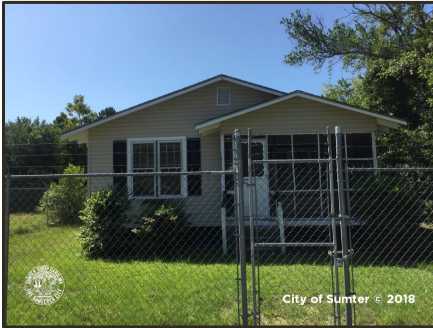
Photograph 1 Bates Example of "Good" Condition Property
