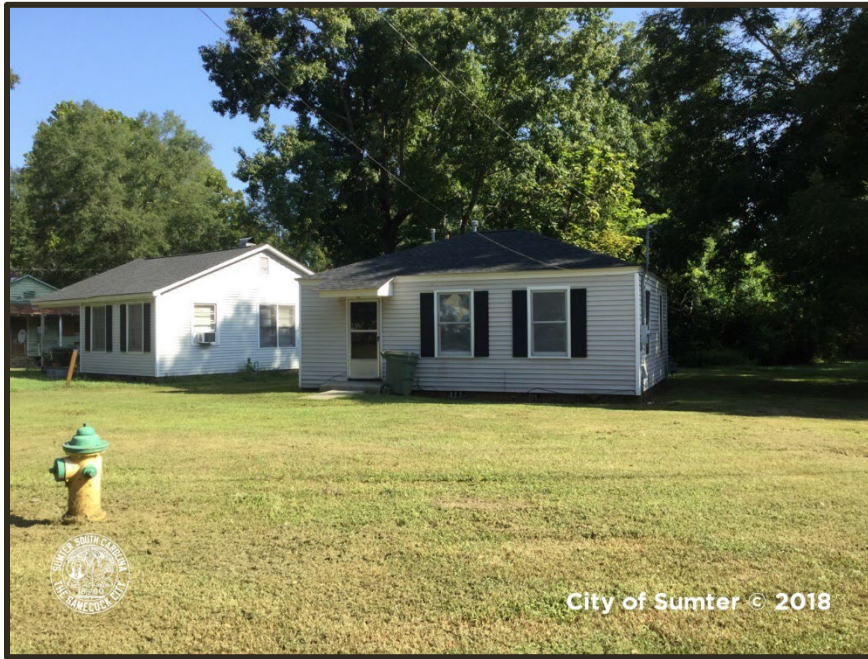
Photograph 30 Magnolia-Harmony Example of "Good" Condition Property
