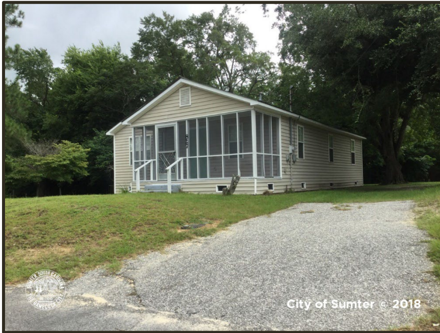
Photograph 43 Palmetto Park Example of "Good" Condition Property
