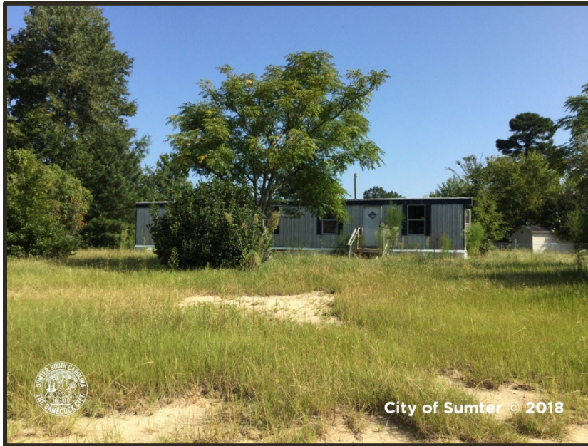
Photograph 24 Lemira Example of "Poor" Condition Property
