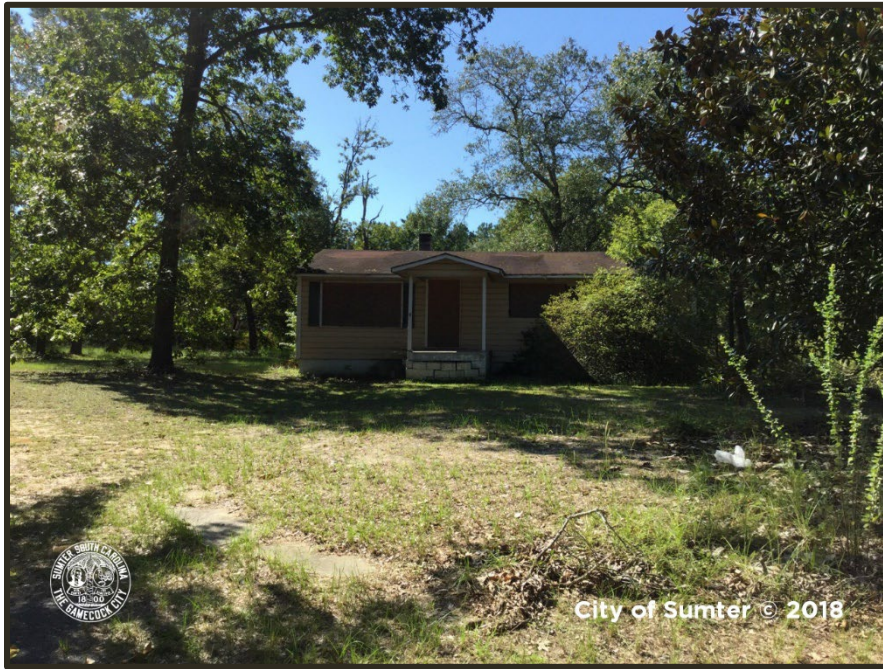
Photograph 56 Spectrum Example of "Poor" Condition Property
