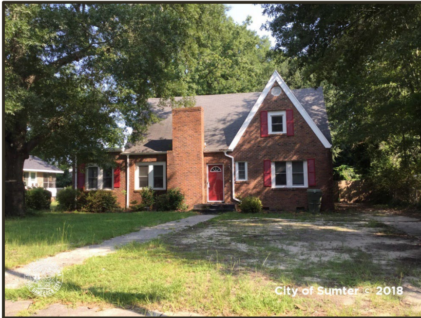
Photograph 26 Loring Example of “Good” Condition Property
