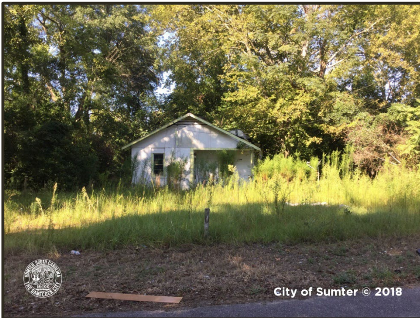
Photograph 48 Savage Glover Example of "Hazard" Condition Property
