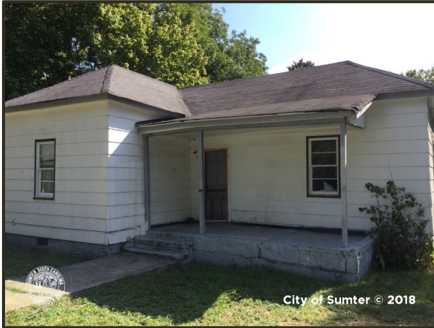
Photograph 58 Stone Hill Example of “Fair” Condition Property
