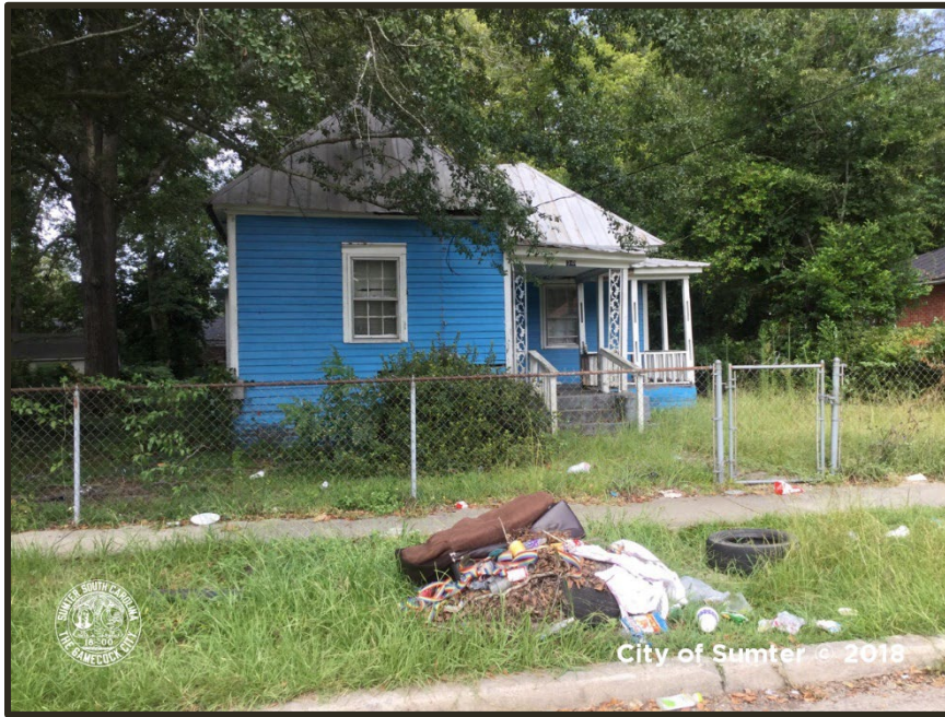
Photograph 7 Birnie Example of "Poor" Condition Property
