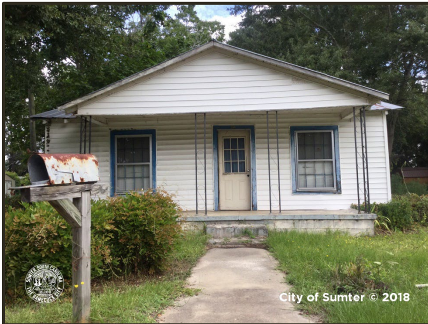
Photograph 447 Palmetto Park Example of "Fair" Condition Property
