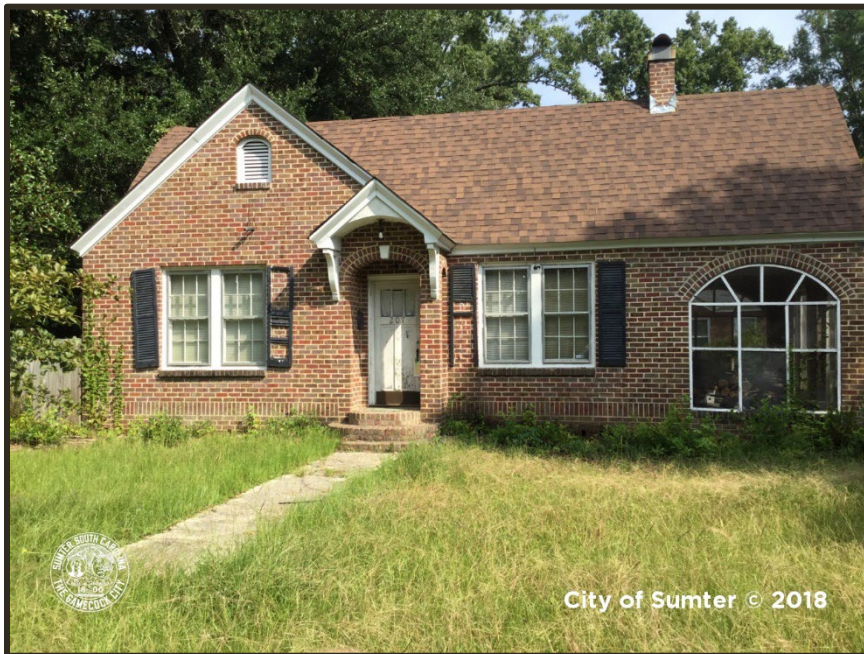
Photograph 27 Loring Example of “Fair” Condition Property
