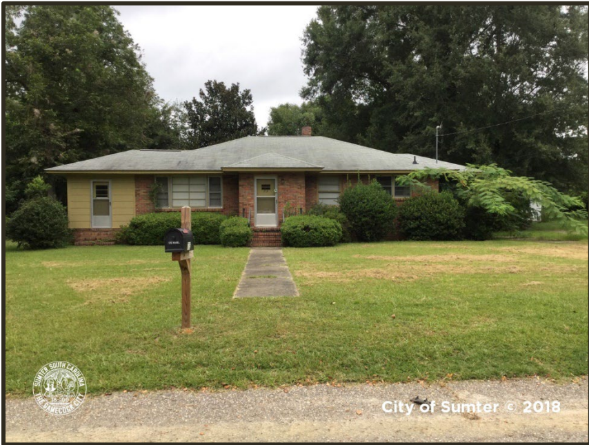
Photograph 49 Second Mill Example of “Good” Condition Property
