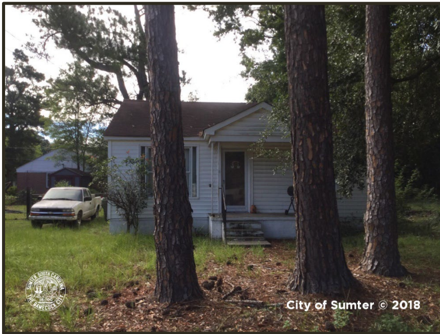
Photograph 16 Folsom Park Example of "Fair" Condition Property
