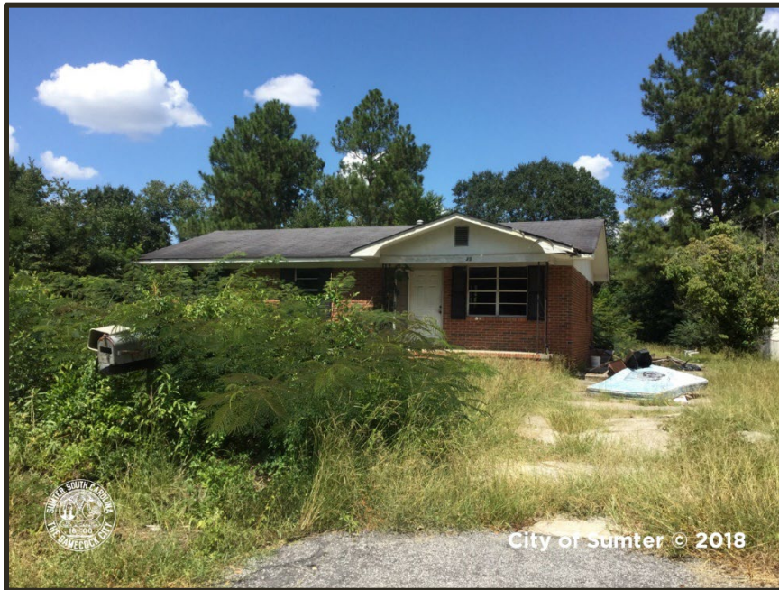
Photograph 57 Spectrum Example of "Hazard" Condition Property
