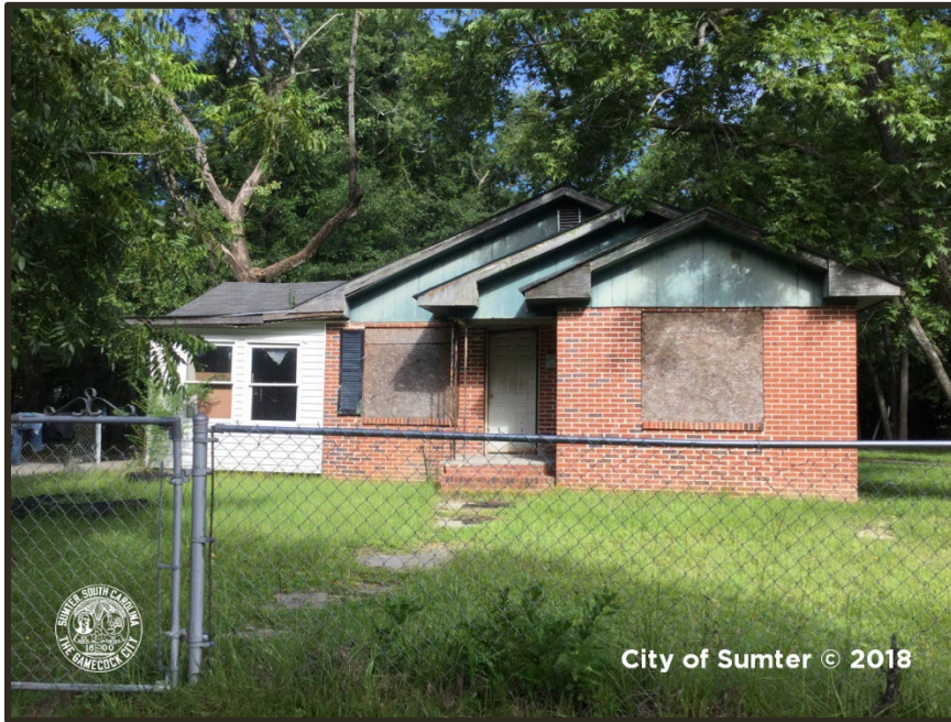
Photograph 17 Folsom Park Example of "Poor" Condition Property
