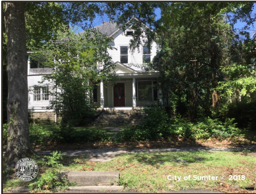
Photograph 21 Hampton Park Example of "Poor" Condition Property
