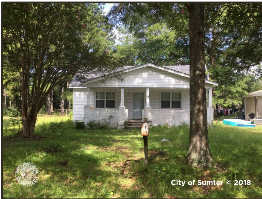
Photograph 379 Morris College Example of "Fair" Condition Property
