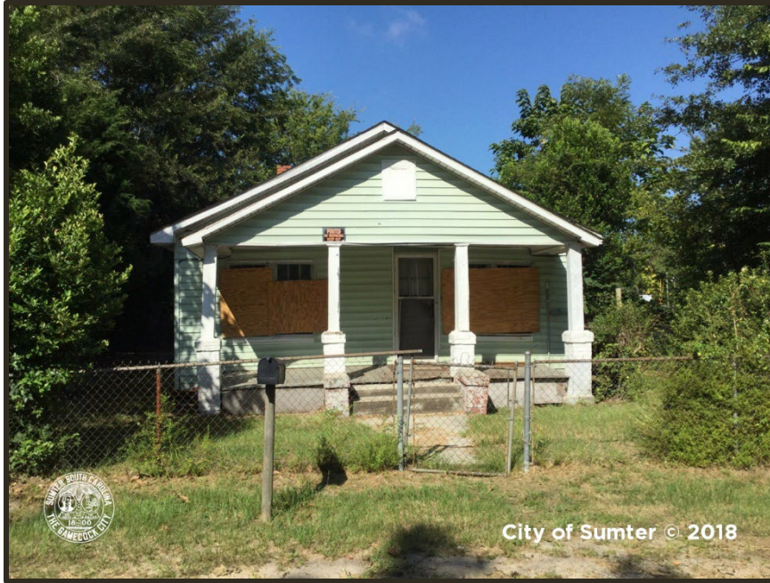
Photograph 59 Stone Hill Example of "Poor" Condition Property
